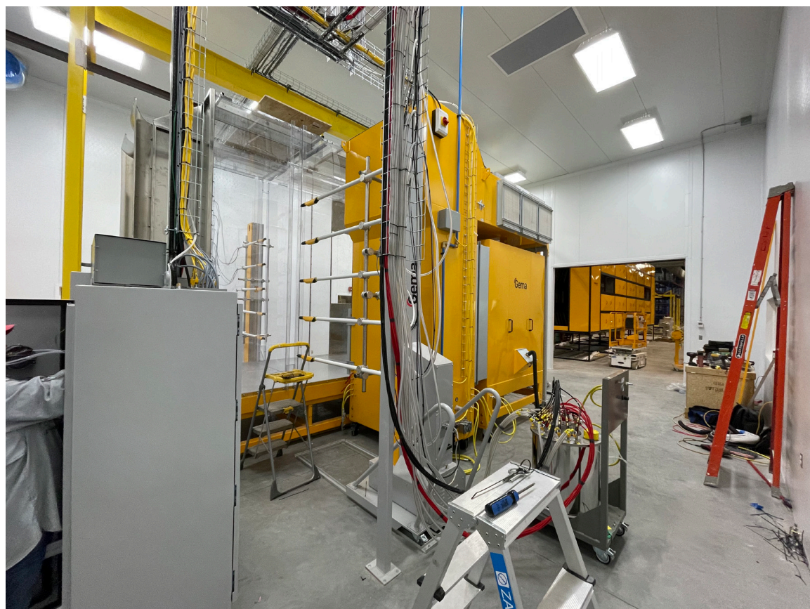
QTG's new Gema paint system enables the company to offer higher-quality finishes, durability, and aesthetic value, while the automated guns allow operators to focus on ensuring a quality process.
